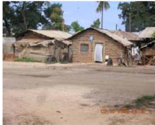
Plate 2: Semi-permanent residential structure at Lilongwe
